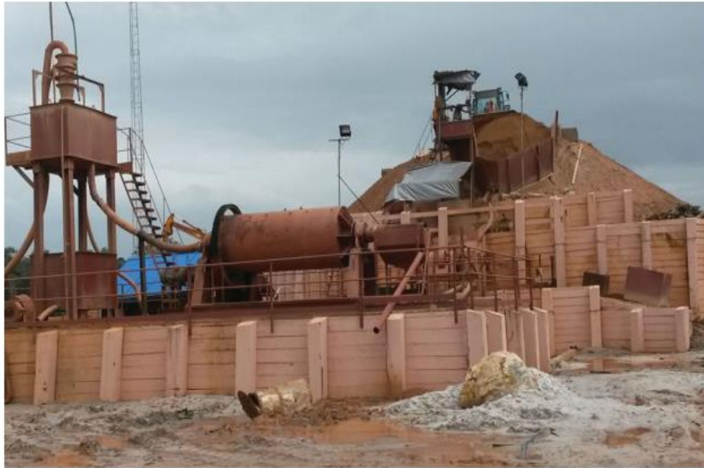
Maripaston gravity concentration plant (photo: R. Finkie).
