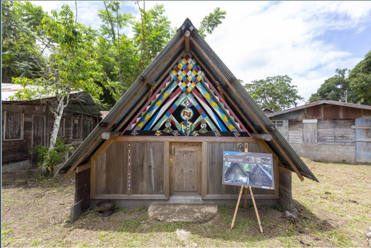
Traditional aluku hut renovated under the "Built Heritage" program. Village of Loka, French Guiana.
