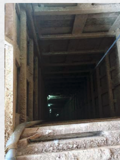
Tunnel operation (Suriname)
